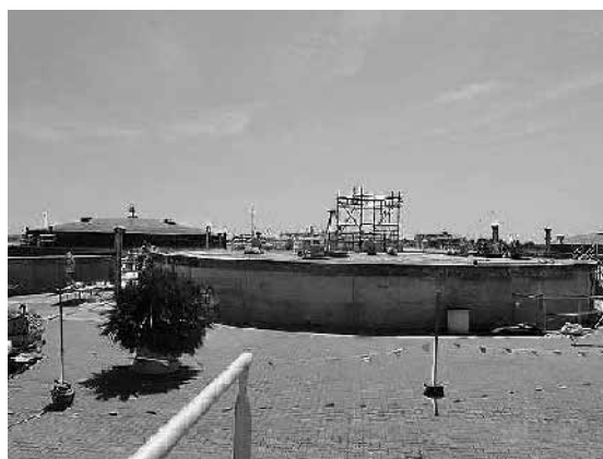
写真1 Glenelg Wastewater Treatment Plant
